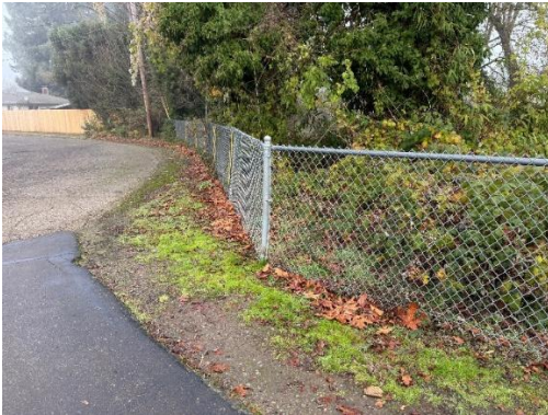
Figure 4 North of the Santiam Street bridge showing steeply sloped canal bank precluding sidewalk construction.
