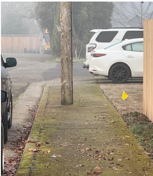
Figure 5 Utility pole placement in sidewalk north of East Carolina Street
