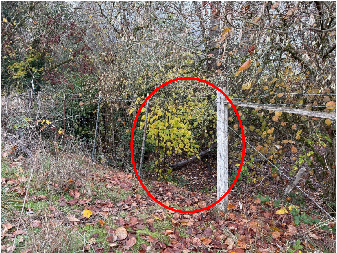
Figure 8 Fence on subject property cut to allow trespass from River Park.
