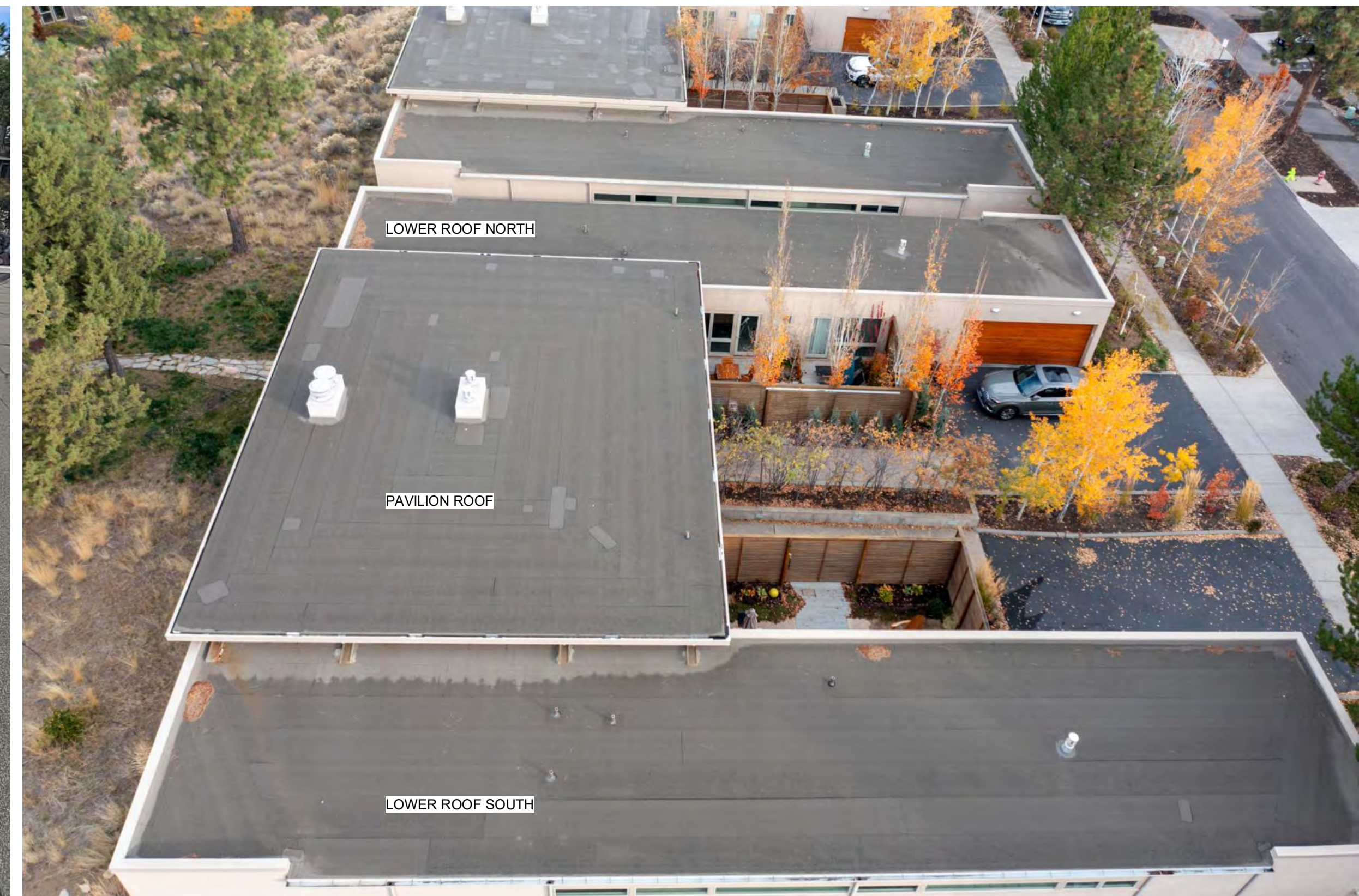
AERIAL VIEW OF BUILDING TYPE A
