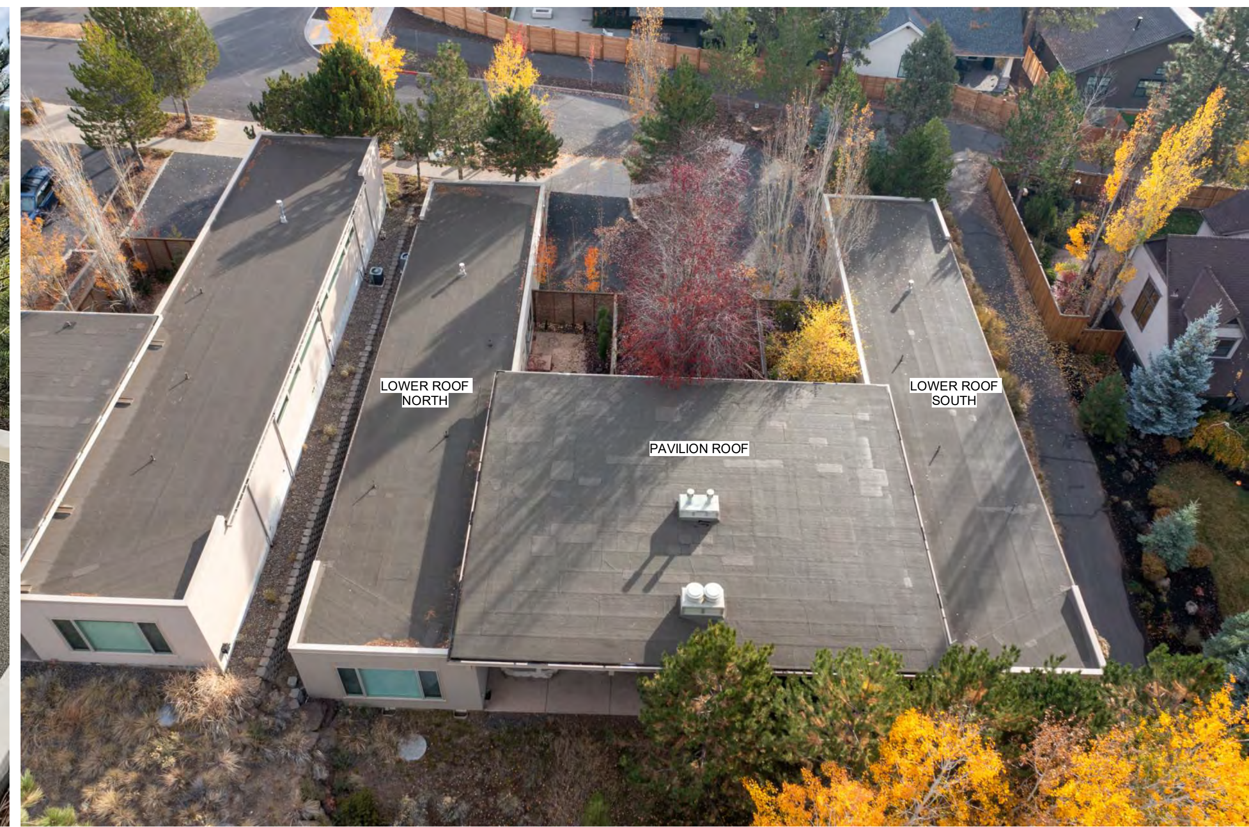
AERIAL VIEW OF BUILDING TYPE A
