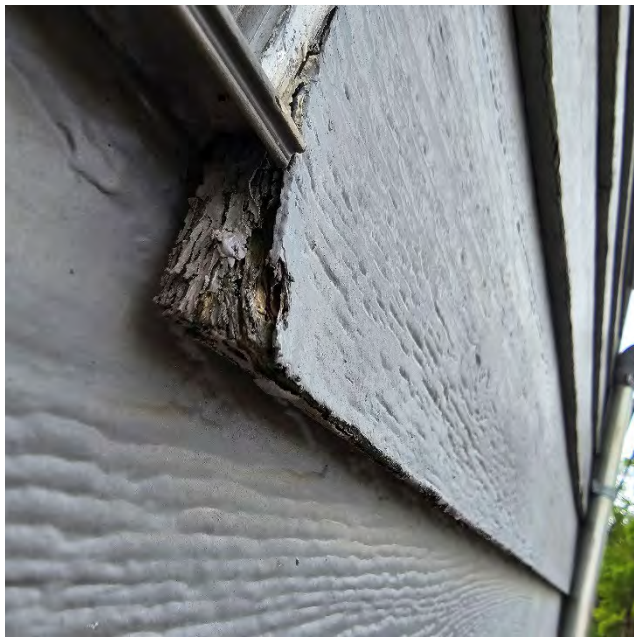
Photo 3.17: Siding edge condition at 2 nd floor door
