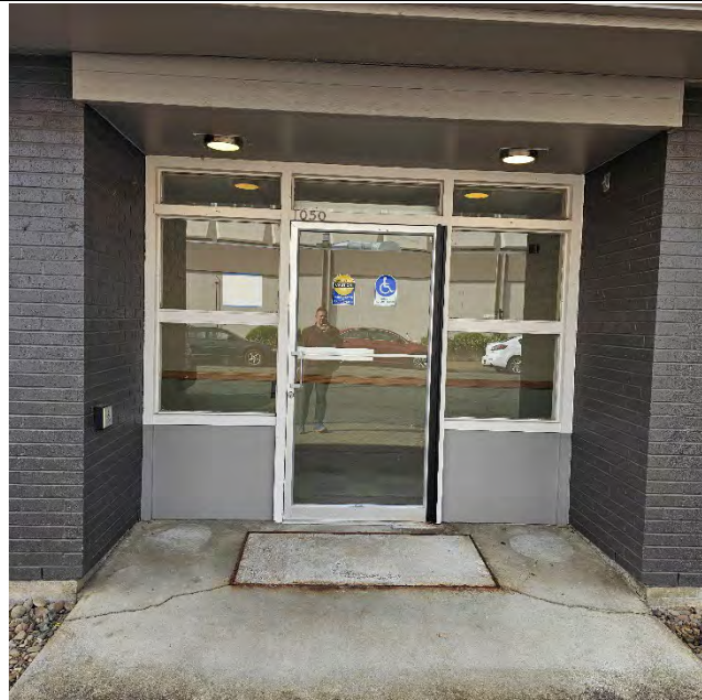
Photo 4.1: Entry siding detail (2249, typ)
