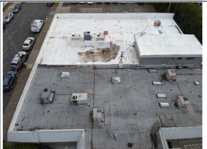
Photo 2.2: West roof overview
