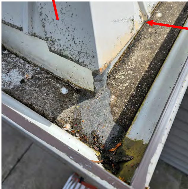
Photo 3.9: Mansard to gutter outside corner condition
