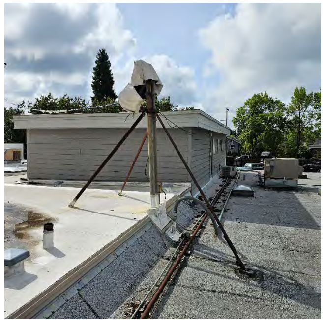
Photo 2.12: Roof weatherhead
