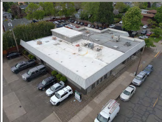
Photo 2.1: East roof overview
