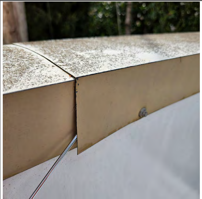
Photo 2.4: Parapet overlap at East roof
