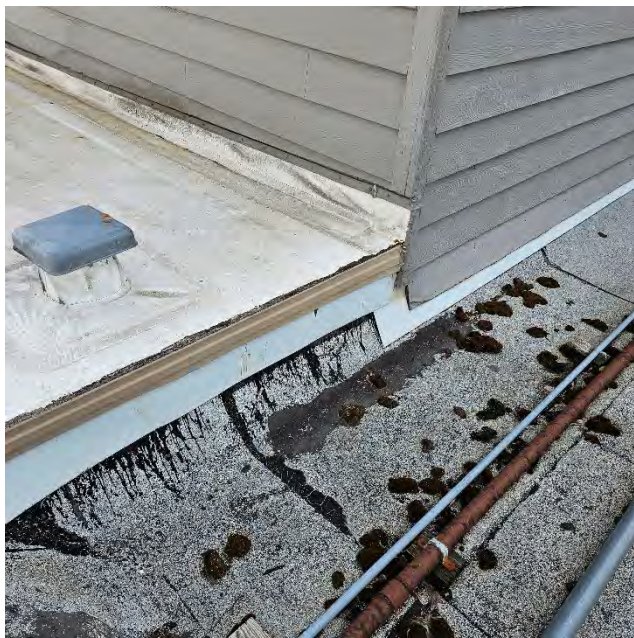
Photo 2.7: East to West roof transition
