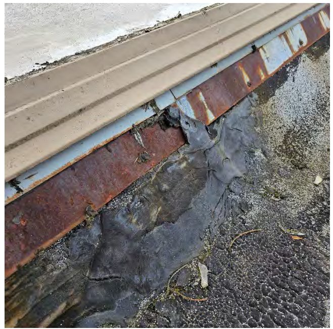
Photo 2.8: Multiple layers of transition flashing
