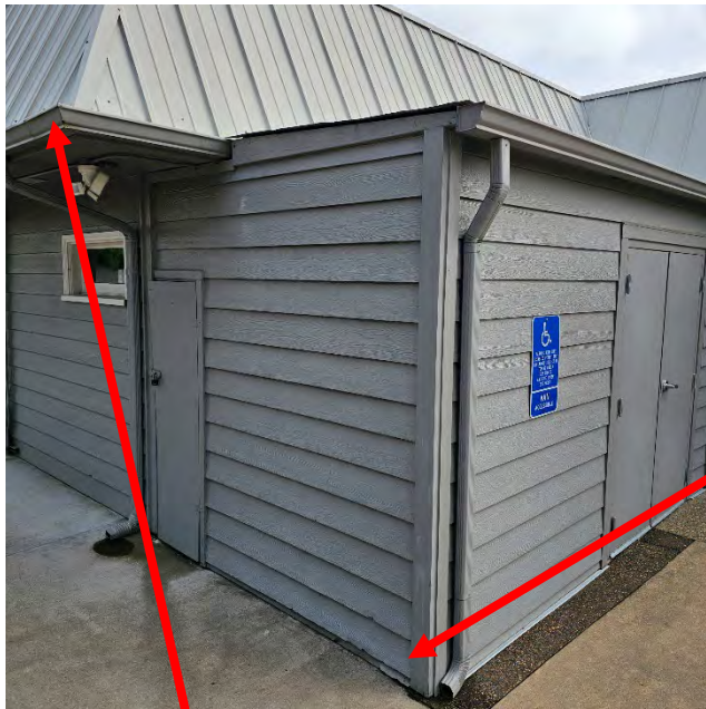
Photo 3.7: Cladding overview at SW corner
