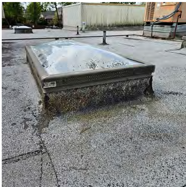
Photo 2.9: West roof skylight
