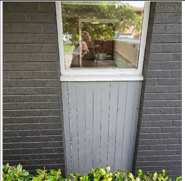
Photo 3.4: Vertical wood siding detail
