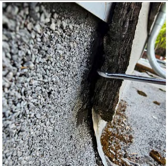
Photo 3.16: Siding edge condition
